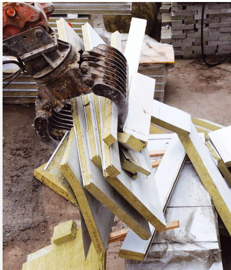
Mobile recycling unit shredding composite panels.
